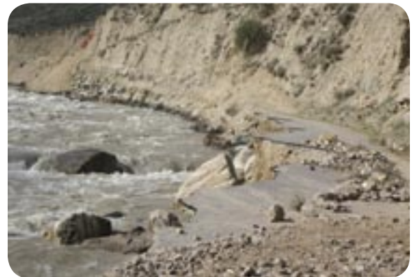
Figure 2.2: Transportation Links Affected by Hydro-Meteorological Hazards
